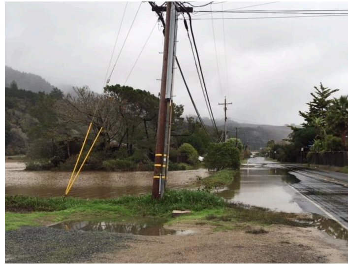
Flooding at a low lying area (approx. 500ft) between Walla Vista and Sacramento Patio along Calle del Arroyo. Photo was taken during a king tide event on November 24, 2015
