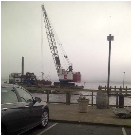
Figure 4.4. Bodega Harbor dredging in 2017. Photo: Cea Higgins.
