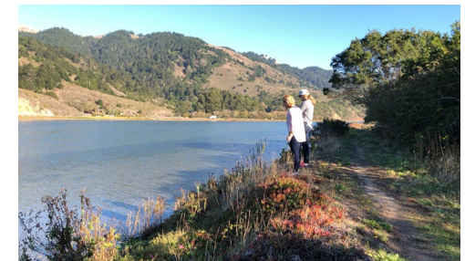
Image 2: Steep eroding shoreline along the eastern span of Dipsea Road.
